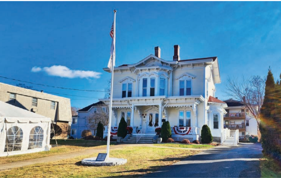
THEY SERVED: This Woonsocket home was renovated and will be used for transitional housing for female veterans. On Monday, Johnston’s OSDRI reopened the Woonsocket Home for Veterans in honor of Marine Corporal Andrea T. Ryder. (Photo courtesy OSDRI)
